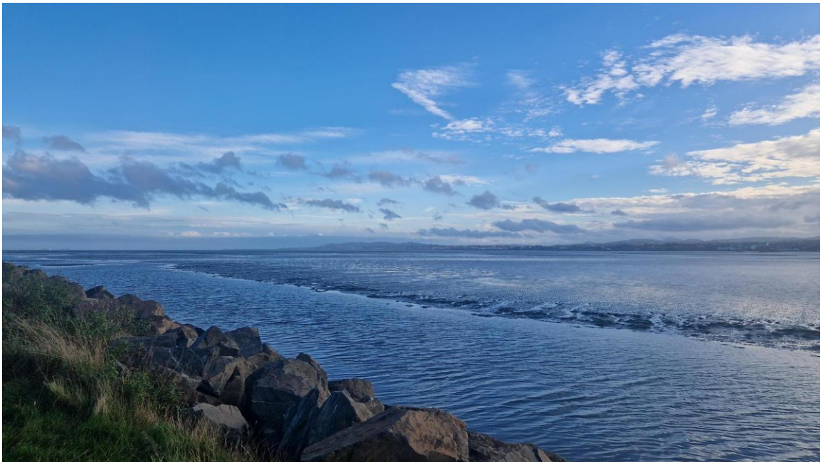
Plate 2 Channel which runs alongside coastline rock revetments within the intertidal area
