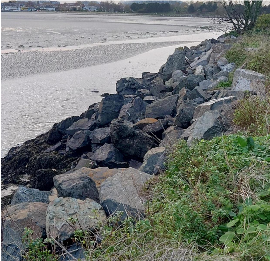
Plate 3 Example of the rock revetments in proximity to the proposed which dominate the coastline of the Poolbeg Peninsula
